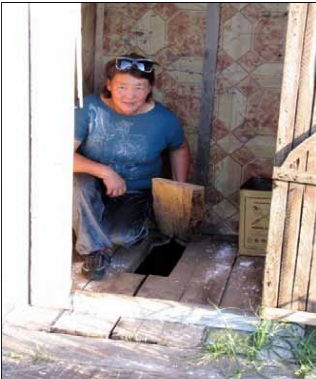
Dry pit latrine with retractable wooden lid-cover constructed within a few days of triggering in villages in Zuunkharaa Sum in Mongolia
